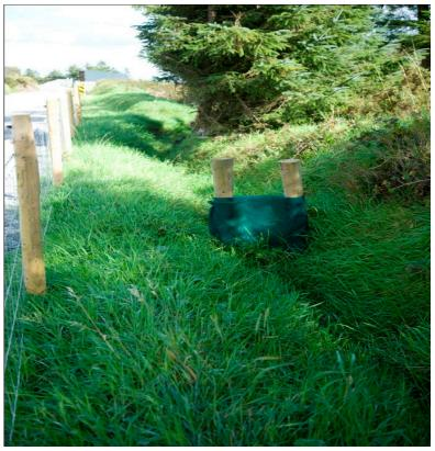
Figure 4-5: Silt Trap across Grassed Swale
