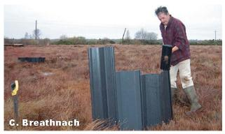
Plate 4-1: Plastic pilling being installed within IPCC bog
